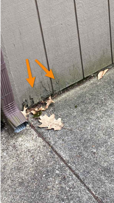
Siding at Basement Patio
