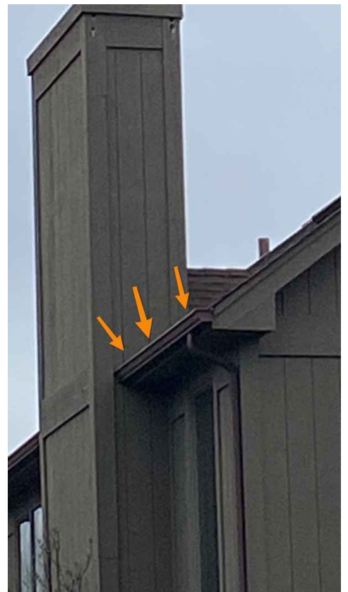
Missing Chimney Flashing
