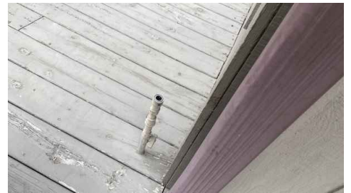
Gas Line Protruding Through Deck Flooring
