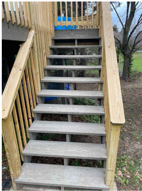
Rear Deck Stairs & Railings
