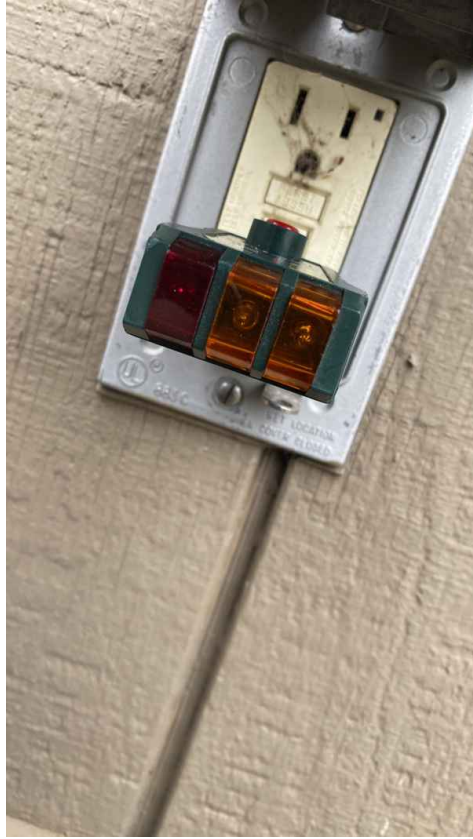
Receptical at Rear Deck
