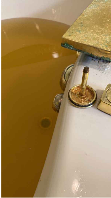
Non-Operational Drain in Jet Tub
